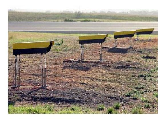
The Precision Approach Path Indicator (PAPI) is a crucial equipment of the Airfield Ground Lighting for a safe approach to the runway even if the airports are equipped with ILS.
